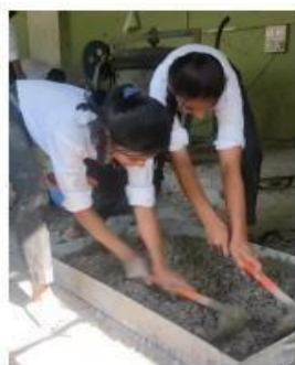
Mixing of Concrete
